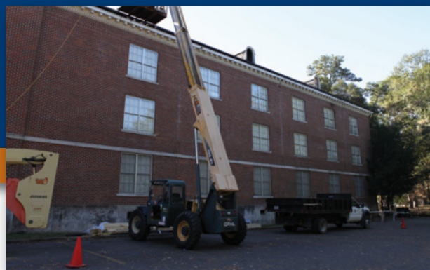
Renovations to Cottingham Hall's roof
